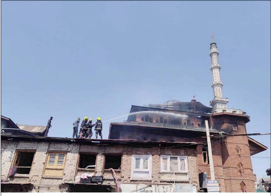
A mosque engulfed in flames in Bagh-e-Dilawar Khan area on Friday in downtown Srinagar. The fire damaged a major section of the mosque as fire tenders were pressed in to douse the flames. UNI
